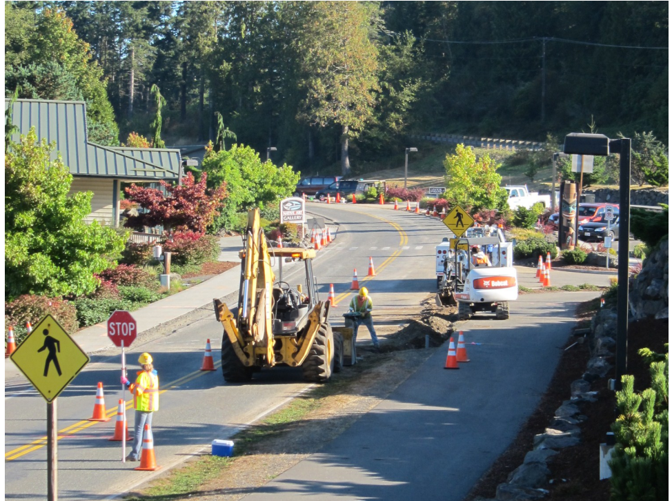
Flaggers controlled one-lane traffic on Old Blyn Highway as crews widened the street to prepare for concrete curbs to be poured.
