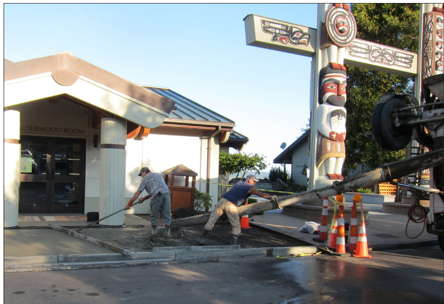
Workers pour and smooth the new concrete in front of the Community Center
