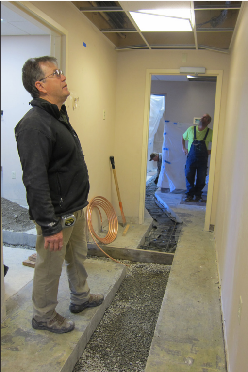
Contractor Jack Grinnell (Prince) surveys the situation during the one-week closure of the Dental Clinic, when the concrete floors were opened to add piping for water and air to each exam room.
