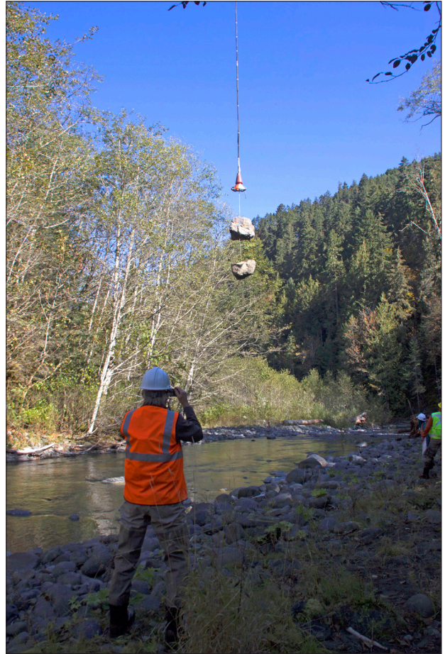
Habitat Biologist Hilton Turnbull watches as large boulders are placed onto the logjam by helicopter
