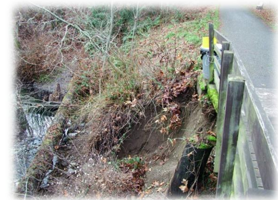
Erosion undercutting the Railroad Bridge
