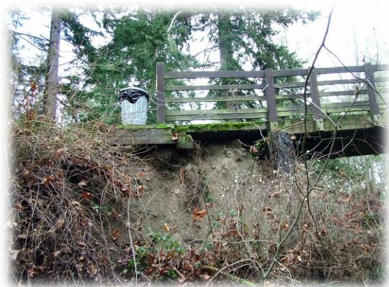
Undercutting at the west end of the Railroad Bridge
