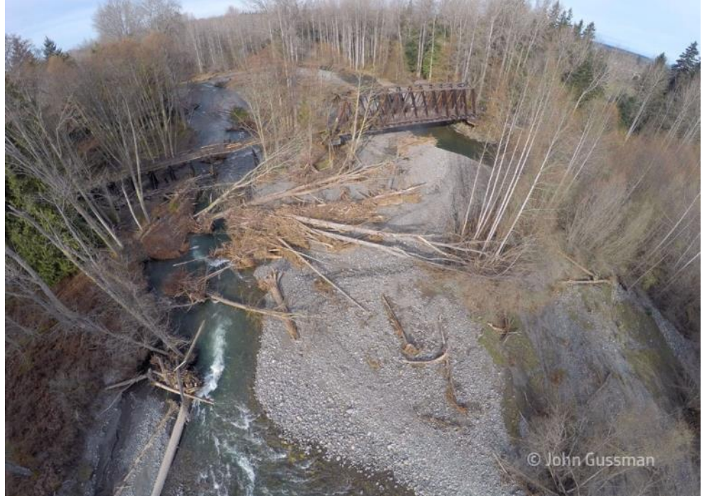
Aerial of the river showing the west (left) side of the bridge after it was damaged, and the large channel flowing under it.
