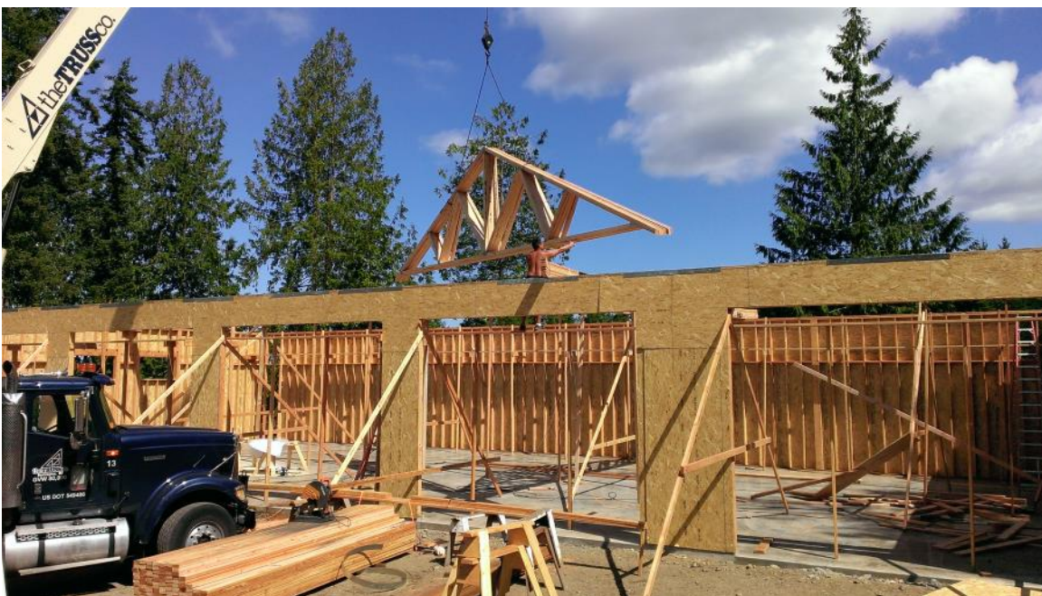
The bus barn shown as the roof trusses are being placed by a giant crane.
