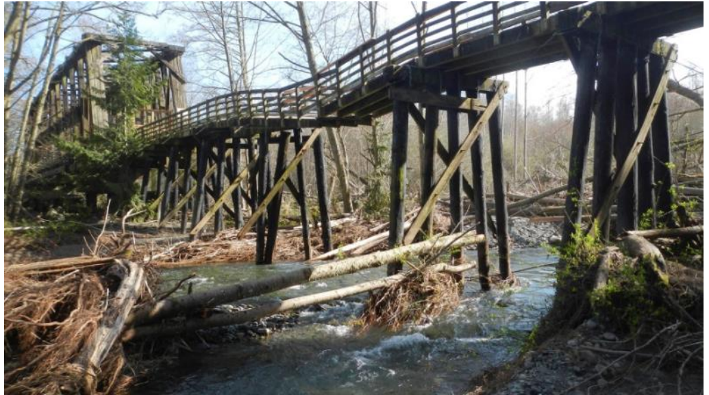
Above, BEFORE: This photo shows the damaged trestle after the February floods. Below, AFTER: This photo shows the new span, which replaced 185 creosote pilings to allow better access for migrating salmon.
