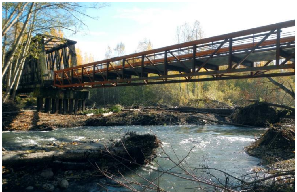
Above, BEFORE: This photo shows the damaged trestle after the February floods. Below, AFTER: This photo shows the new span, which replaced 185 creosote pilings to allow better access for migrating salmon.
