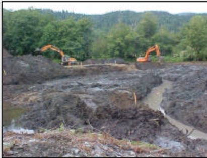
Early stages of construction
