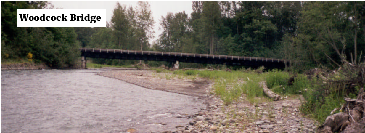
Photo 19: Woodcock Bridge, located at RM 3.3, has a span of 405 ft. This bridge cuts off access to the historic floodplain, constricts the channel migration zone, and causes sediment deposition upstream of the bridge. Photo taken 5-20-98.
