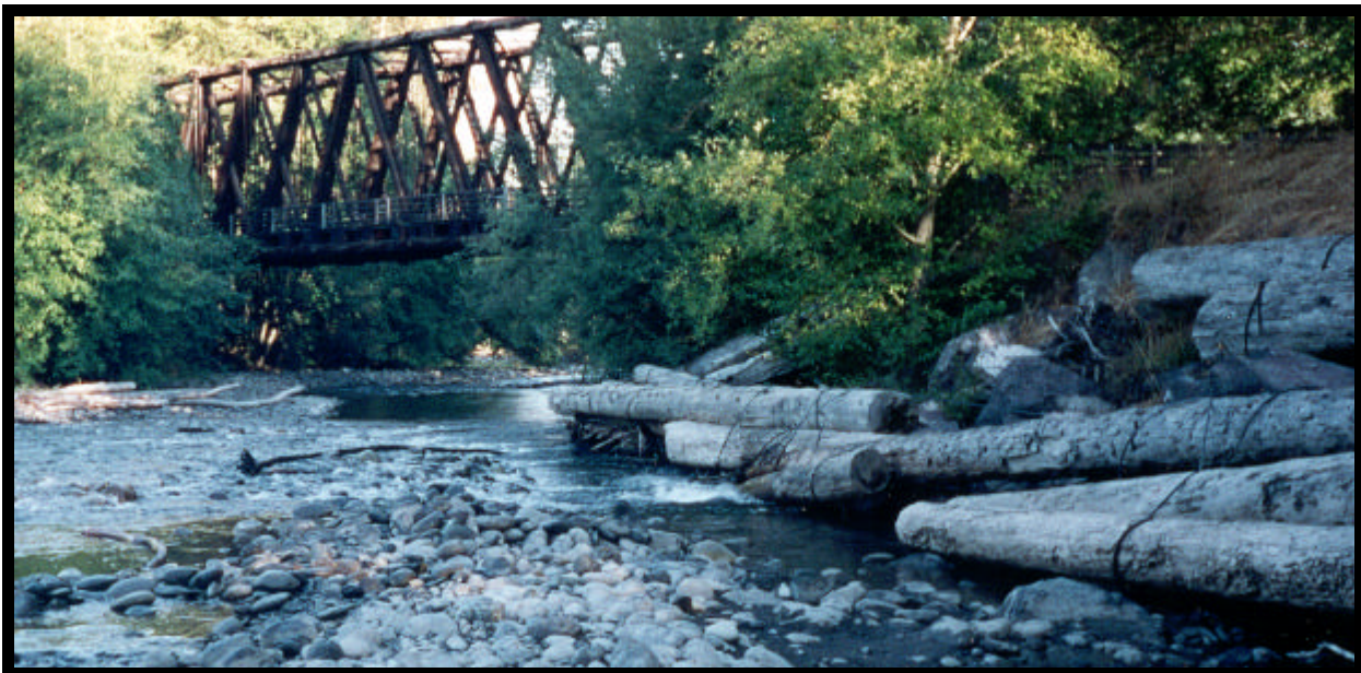
Photos 16: Five bridges cross the lower Dungeness River. The Railroad Bridge (RM 5.7) is heavily used for recreation and a newly developed River Center was built on the east side. A dike (built in 1961) and recently added cabled logs (visible at right) have been built to protect the new River Center. While the bridge does not constrict the active river channel, the dike does cut off the east floodplain.
