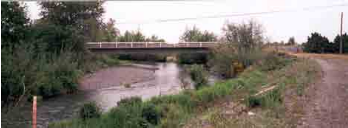
Figure 2. Looking downstream at Schoolhouse Bridge from Corps levee in May, 1998.
