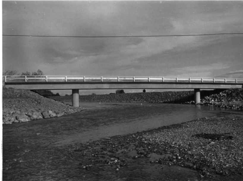
Figure 6. View downstream showing Schoolhouse Bridge after completion of construction and channel widening in 1964. Note the broad, flat configuration of the river channel bottom following channel widening. The Army Corps of Engineers flood-control levee is present on the east terrace. Photograph courtesy of the Clallam County Road Department.
