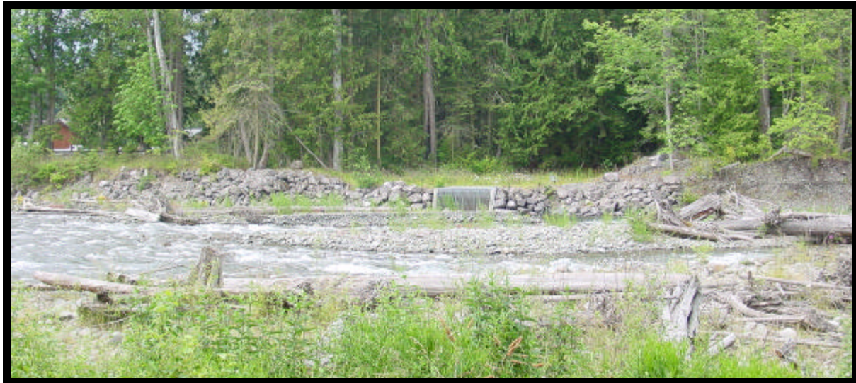
Photo 28: In addition to bridges and levees, irrigation diversions and bank protection as shown above are common features along the study reach. Bank protection does impact natural processes by preventing natural channel migration and recruitment of large woody debris. In some areas, rock has been placed on the banks of river terraces that are hundreds to thousands of years old. Although erosion of river terraces can be a natural process, the erosion can be accelerated by human impacts to the river. In some cases, protection of terraces can be considered a mitigation for one or more human impacts. Photo taken 6-28-01.
