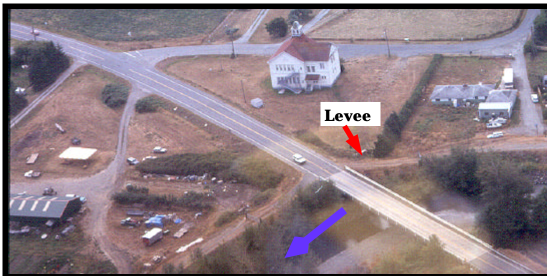
Photo 25: Schoolhouse Bridge (RM 0.8) is located at a natural constriction formed by glacial knobs. The river has likely flowed through these knobs for thousands of years. Prior to levee construction upstream of the bridge, flood flows would spill over river banks onto the floodplain. A portion of these flows would enter Meadowbrook Creek which flows into Dungeness Bay. Today, levees force all the water to pass under Schoolhouse Bridge. Photo taken 9-10-98.
