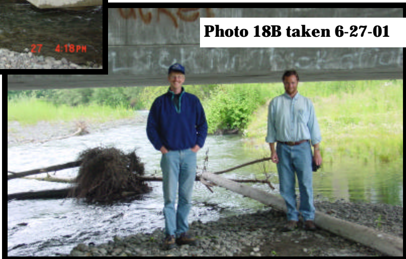
Photos 18A and 18B: The new Burlingame Bridge was built with an increased opening of 430 ft and no longer cuts off access to the wooded floodplain. During a recent site visit, woody debris and gravel bar deposition was observed under the bridge. Future changes in channel bed elevation and woody debris accumulation should be monitored to ensure the safety of the bridge.
