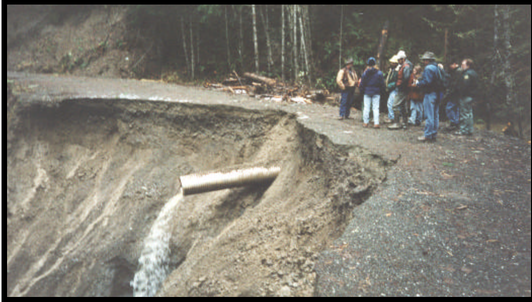
Photo 15: Numerous human impacts have affected the Dungeness River throughout the watershed. Several logging roads have been constructed in the upper watershed. Rainfall runoff can concentrate where a drainage crosses these logging roads. This concentrated flow can accelerate erosion processes including landslides such as shown here. These types of landslides can be a significant source of fine (silt and clay) sediment to the river channel. While these sizes of sediment do not cause channel change, they can increase turbidity in the river channel affecting fish feeding and spawning. Photo taken 5-17-00.
