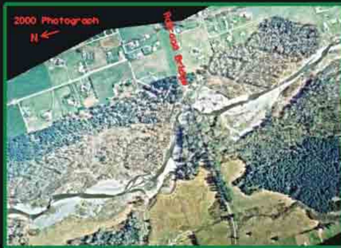
Figure 26. Bank erosion in the section of Reach 3 near Railroad Bridge. Eroded portions of the bank are for the time intervals between aerial photographs as shown.
