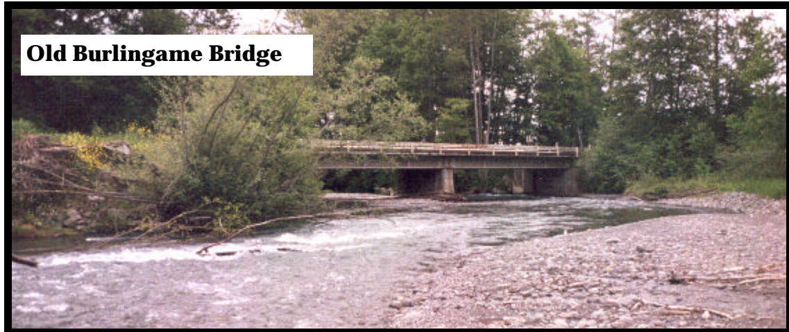
Photo 17: The Burlingame Bridge on Old Olympic Highway (RM 4) was replaced in 1998-99. The old bridge had a span of 130 ft which constricted the active river channel and cut off access to side channels and floodplain. Photo taken 5-21-98.
