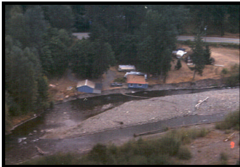
Photo 30: While development in the floodplain can impact natural processes, the river can also impact development in the flood plain (such as at RM 9.2 in photo 30). Management decisions to implement river restoration have the tough task of balancing natural river processes with the protection of existing infrastructure. Photo taken 9-10-98.
