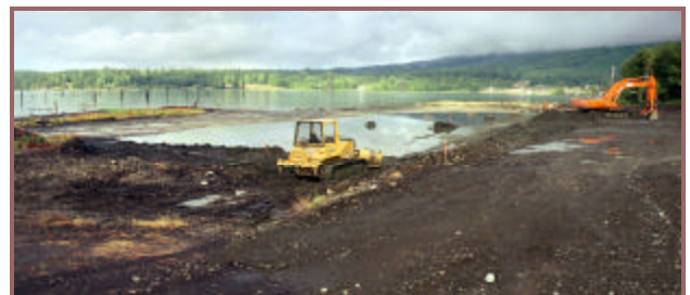
Excavation of the log yard pier and fill
