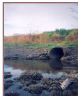
Salmon blocked access to creek
