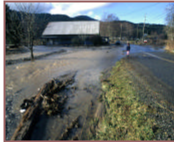
1997 Flooding on Old Blyn Highway
