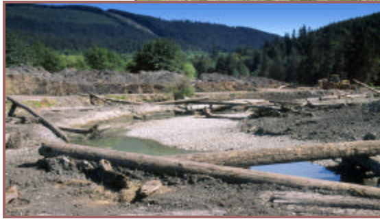
Newly cut channel with spawning gravel, LWD and plantings
