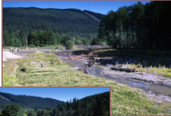
Newly cut channel with spawning gravel, LWD and plantings
