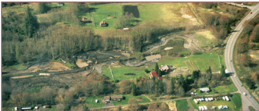
IN PROCESS: Aerial of newly completed channel upstream of Highway 101 —March, 2003
