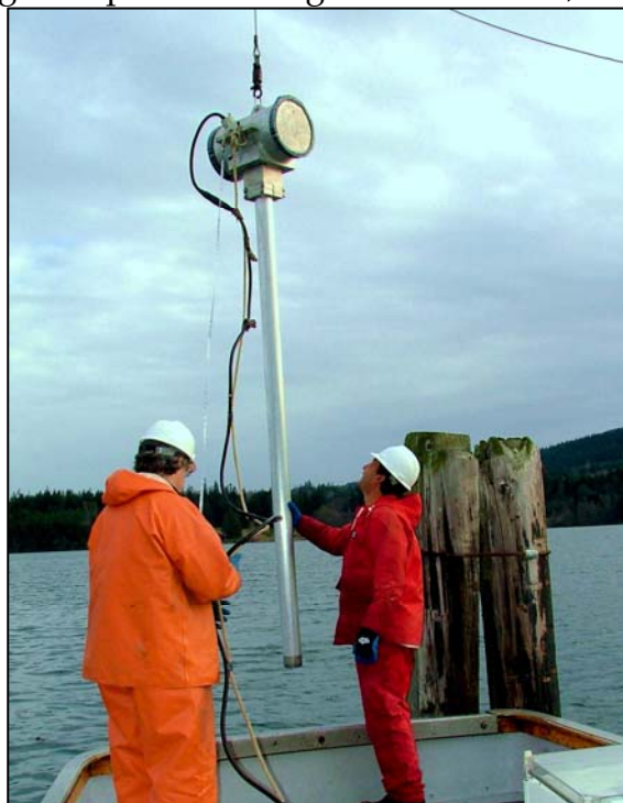
Figure 2.2. Electric vibratory hammer in Sequim Bay.
