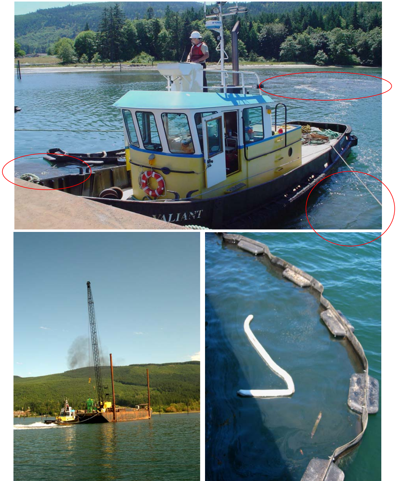
Figure 4.2. Piling removal activities: (a) sediment plumes associated with tug boat movements; (b) tug boat prop wash (c) creosote sheen following piling removal.
