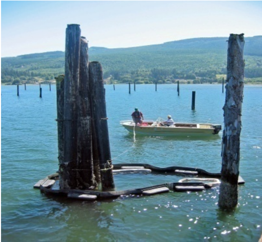
Water quality monitoring during the removal of creosote-treated pilings (Dave Shreffler)
