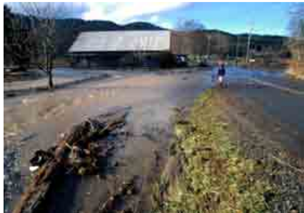
Flood waters overtop Old Blyn Highway, New Year’s Day 1997 (Randy Johnson)
