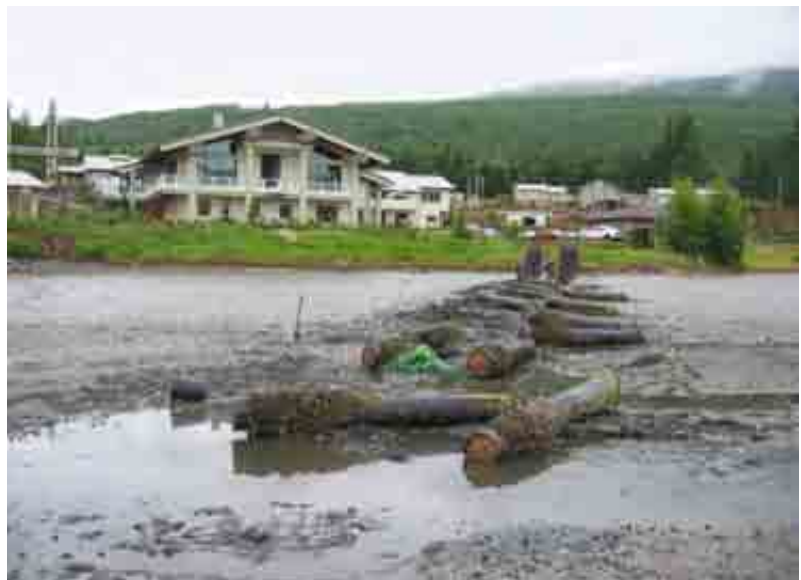
Pilings cut via chainsaw at low tide (Dave Shreffler)
