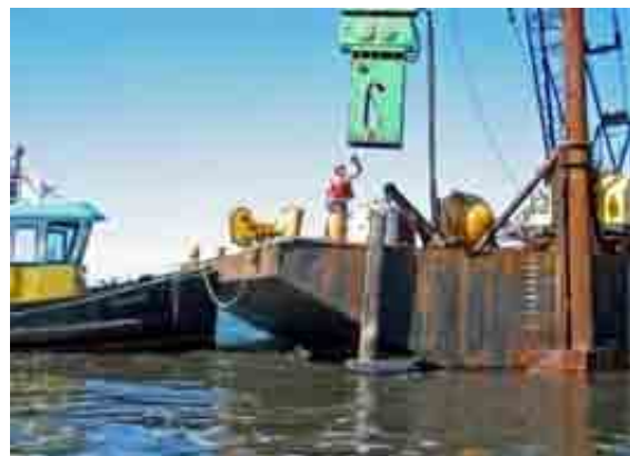
Creosote piling removal via vibratory hammer (Dave Shreffler)
