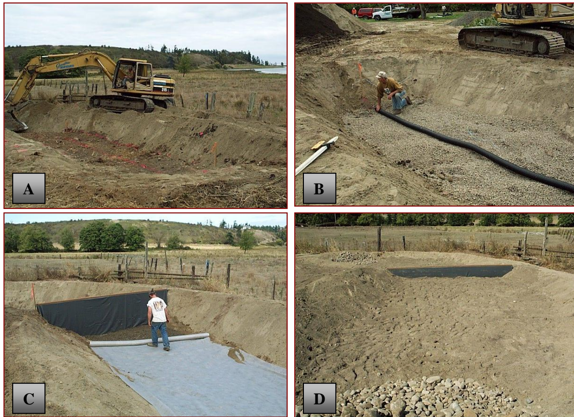
Figure 5. Construction of Twin Biofiltration Cells: (A) Excavation of Twin Cells; (B) Placement of Perforated Underdrain Pipe in Gravel Envelope, (C) Placement of Permeable Landscape Fabric and Impermeable Barrier Between Cells (red arrow), and (D) Energy-Dissipation Rock at Surface Outlet with Layer of Sand and Organic Material
