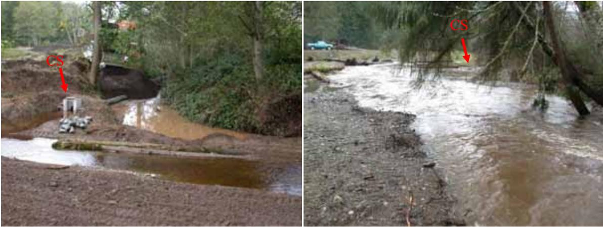
**Figure 1.3.** Left photo: Filling in old JCL channel Oct 25, 2004 (muddy channel in background). Note nursery flow pipe and control structure. New JCL channel flows right to left in foreground. Right photo: Same site during flood on Jan 18, 2005. Note the control structure (CS) (photo center downstream of tree) is almost under water (photos by Byron Rot).
