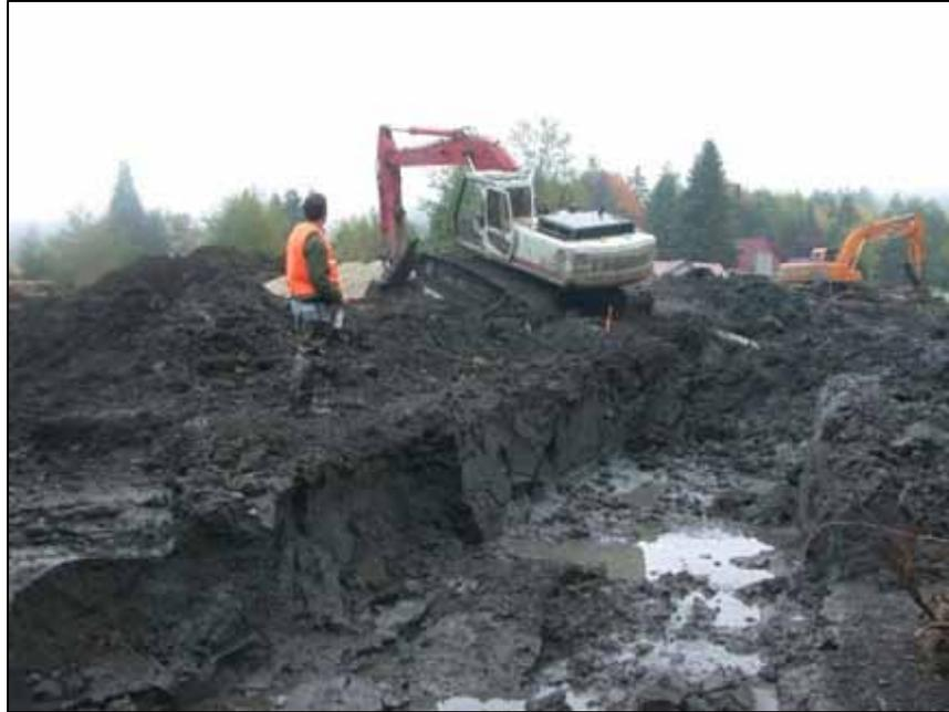
**Figure 2.12.** JCL floodplain construction near 22+00. The new 100 yr floodplain is at the bottom of the trough; the new channel was inset several feet below the floodplain. The surveyor is standing at ground level (October 2002, photo by Byron Rot).
