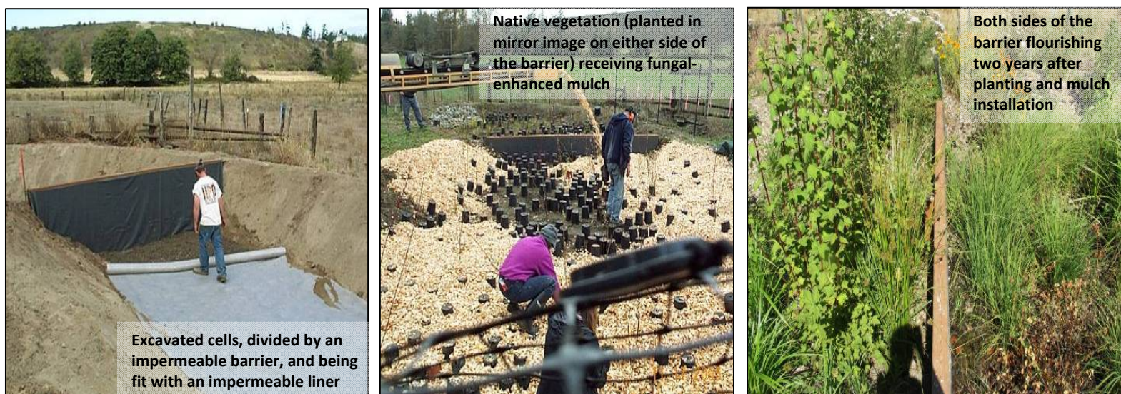
Figure 6. Construction of Mycoremediation Demonstration Site.
