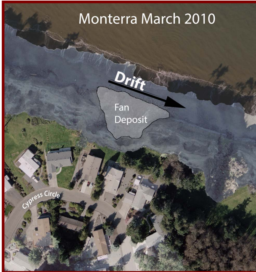
Figure 12: 2010 Aerial images showing the recent rapid recession in the Monterra area of Unit 2. Note the fan shaped debris flow. Additional images of structures close to the bluff crest are provided in Appendix E.
