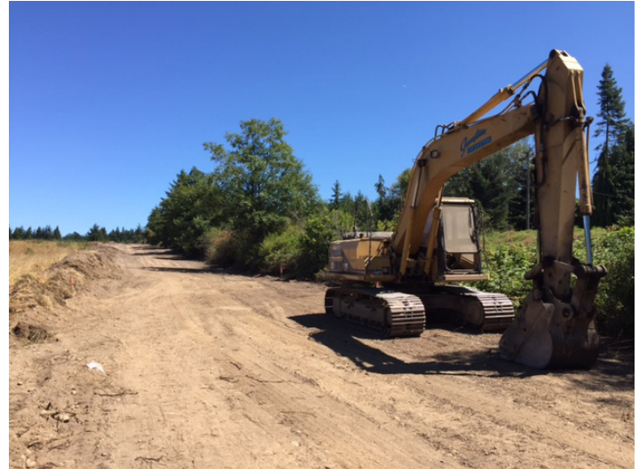
Earth moving for the Olympic Discovery Trail started in July.
