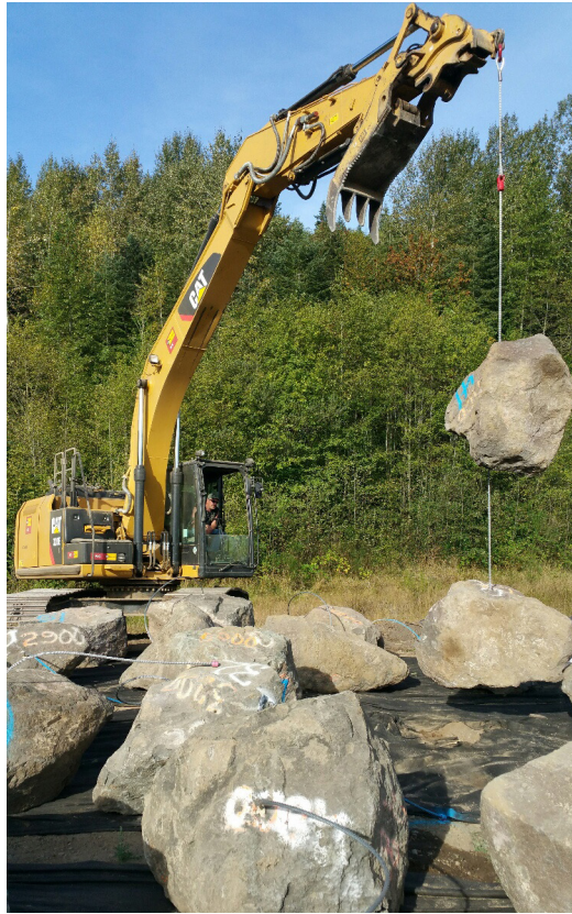
Left, Jamestown Excavating builds the rock-collar anchoring system. Right, engineered log jams on the Dungeness River are circled in yellow.
