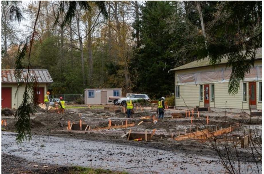
Hiday Concrete crew builds forms for the new River Center foundation.
