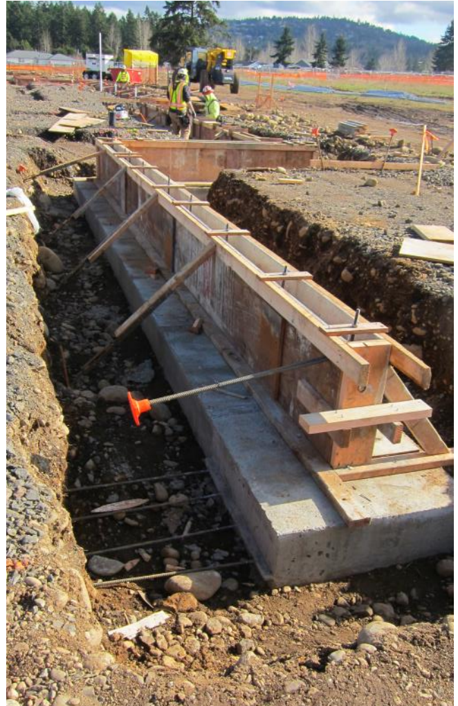
In mid-February, crews were installing forms for the next concrete pour.
