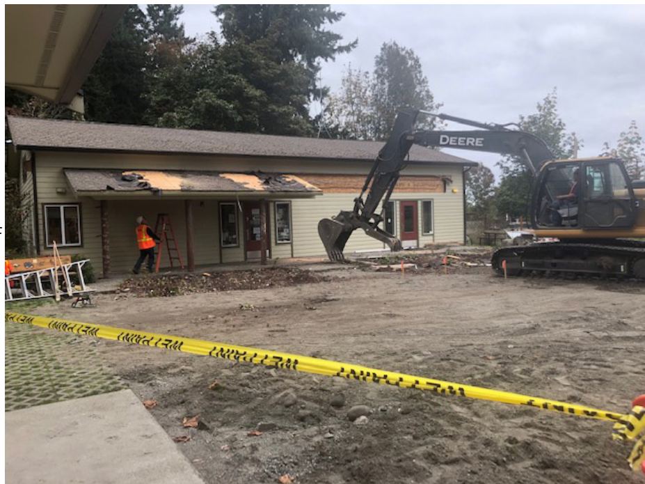
Above, the Dungeness River Center expansion began with JEX removing the permeable parking lot and the shed roofs that would interfere with the new addition to the existing building.
