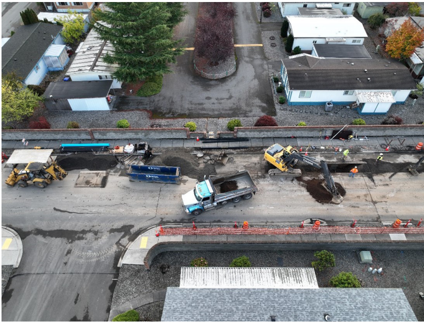
Jamestown Excavating is currently engaged in a large contract for the City of Sequim replacing the Water Main on 7th Street.
