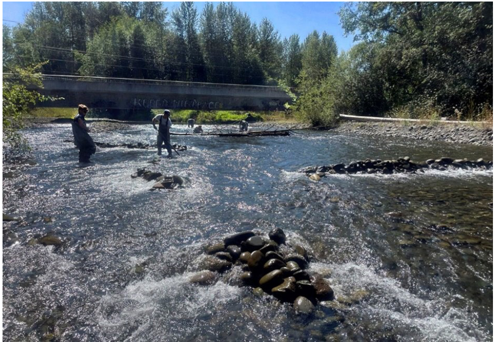
Constructed rock dams help direct fish passage.
