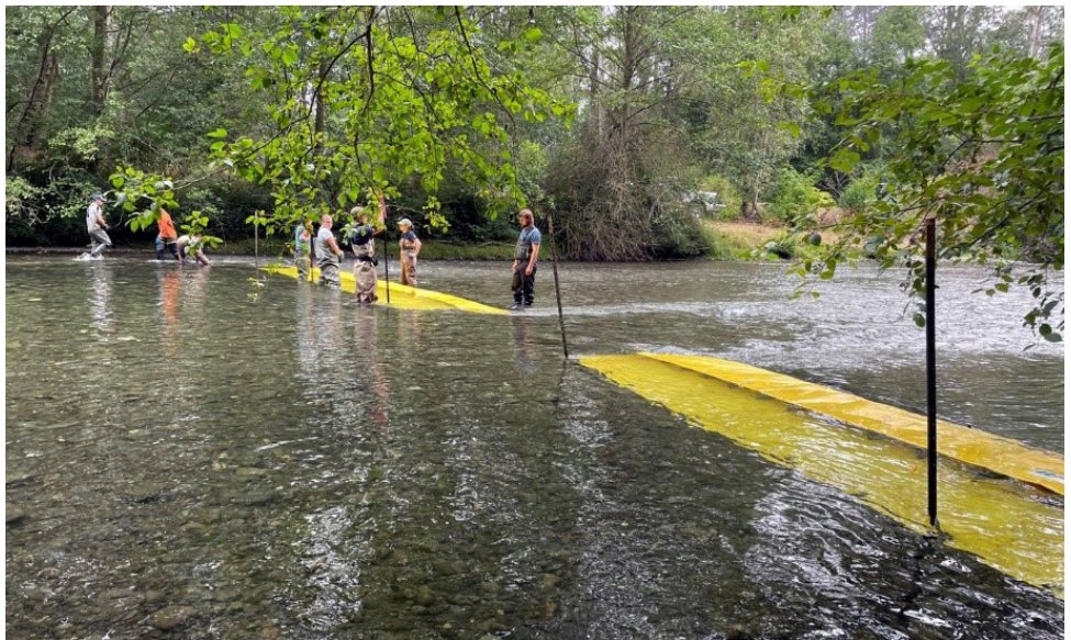
Aqua-dams are installed on wide, shallow riffles in the Dungeness River.
